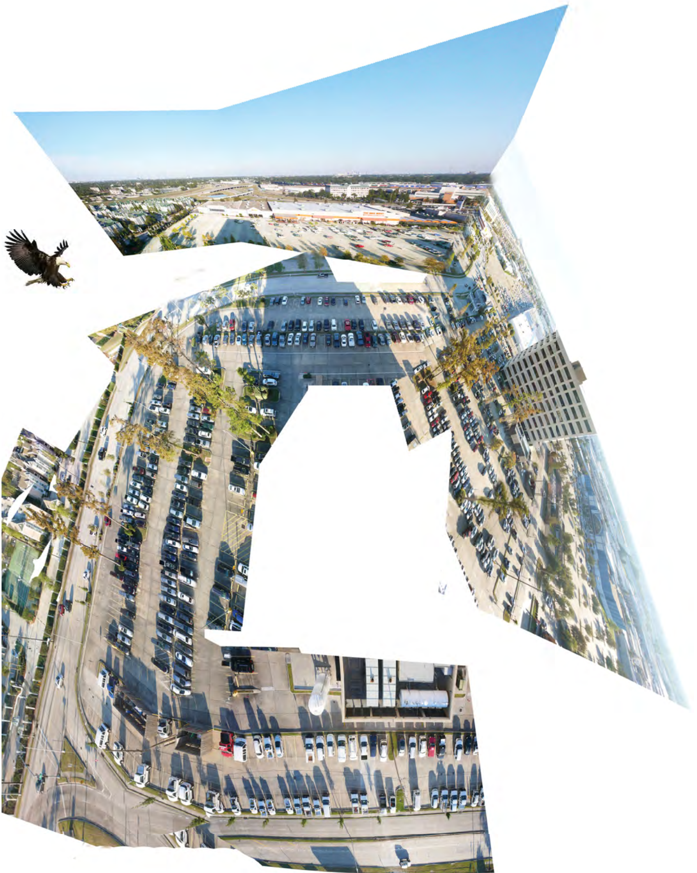
Eagle's eye view of the existing condition of the parking area Joseph S. Yenni building
