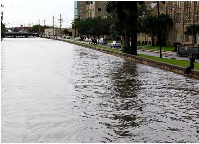
Existing Canal, Wet Weather
