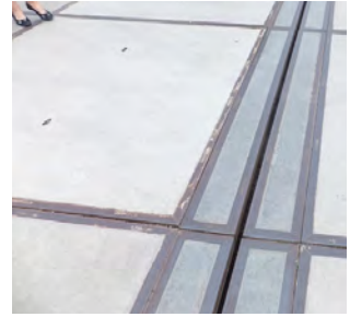
hidden gutter in roadway
