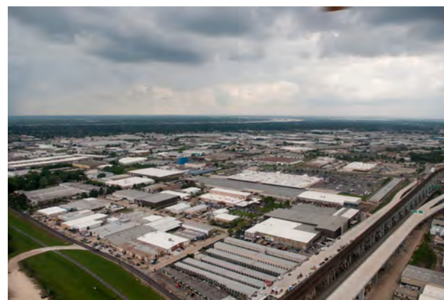
Elmwood District, existing
