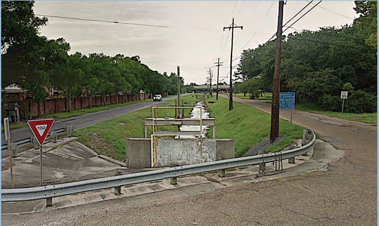
Existing Canal Street Canal
